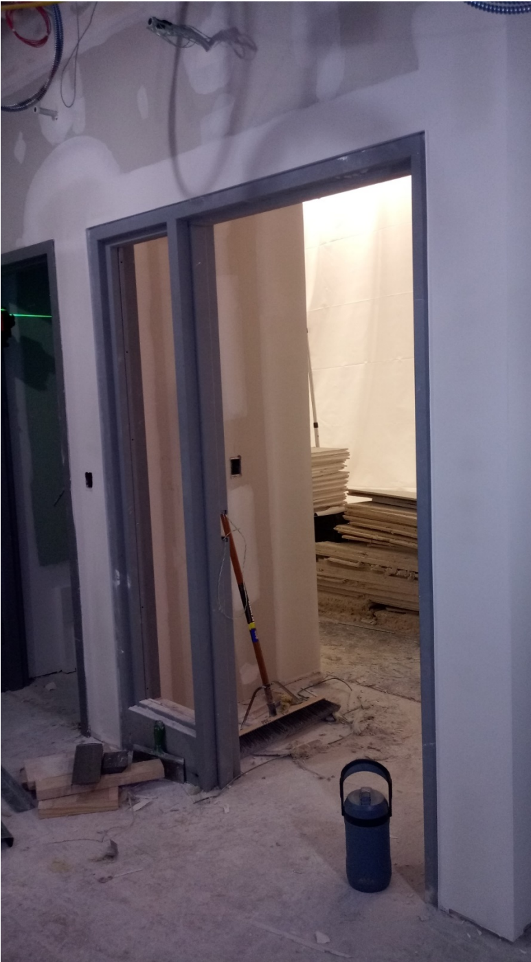
Corridor 118 – Ballistic storefront framing installation.
