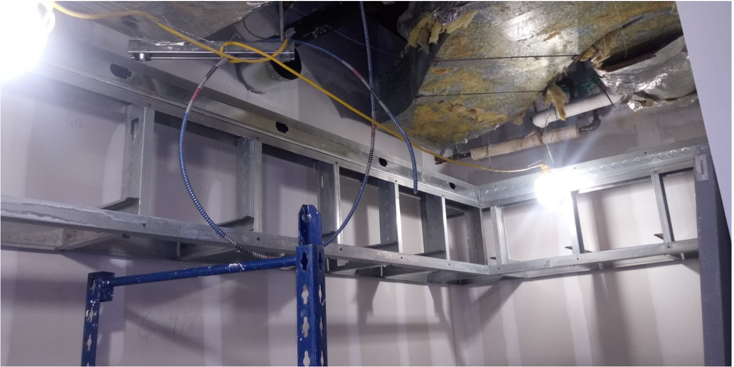
Corr. 118 – Framing above lockers.
