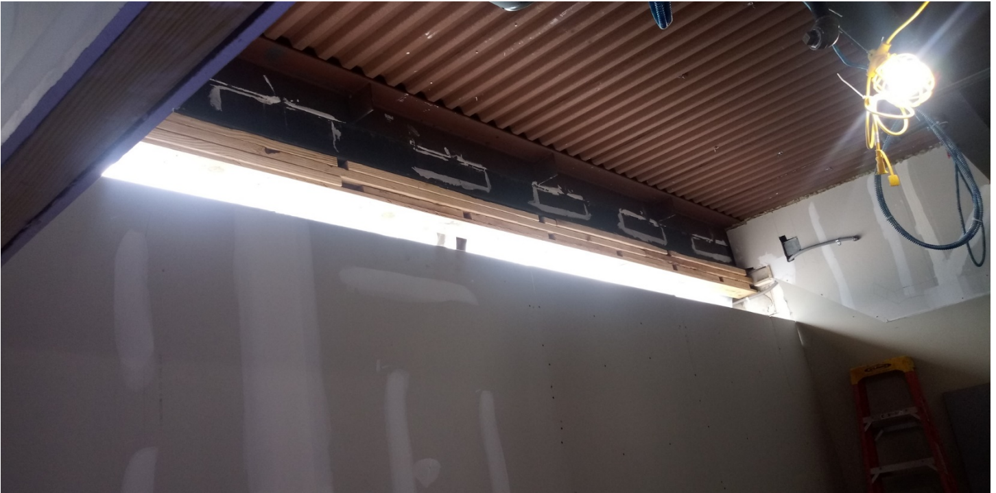
Office 111 – Window demo & blocking installation.
