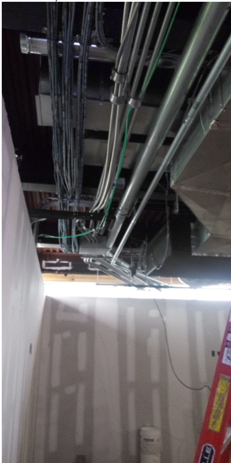
Dispatch 120 – MEP routing / ductwork continues.
